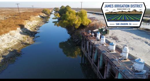
The District ceased diversions the week of December 4, 2023, as the Mendota Pool is currently undergoing maintenance. Pictured above is our main lift station on the James Bypass at Lateral P where three sources of surface water are brought into the District's Main Canal.
